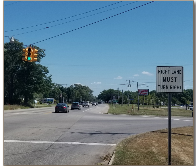
US 31 & M-55 Intersection (lack of sidewalks, crosswalks and signalization)
