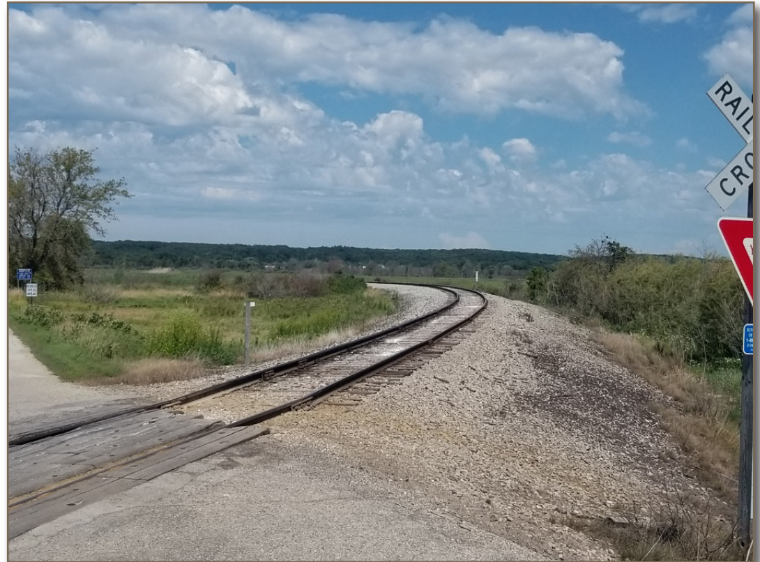
Railroad Track and Bed Vicinity of Penny Park (Railroad Relocation Allows for Conversion to Trail System)
